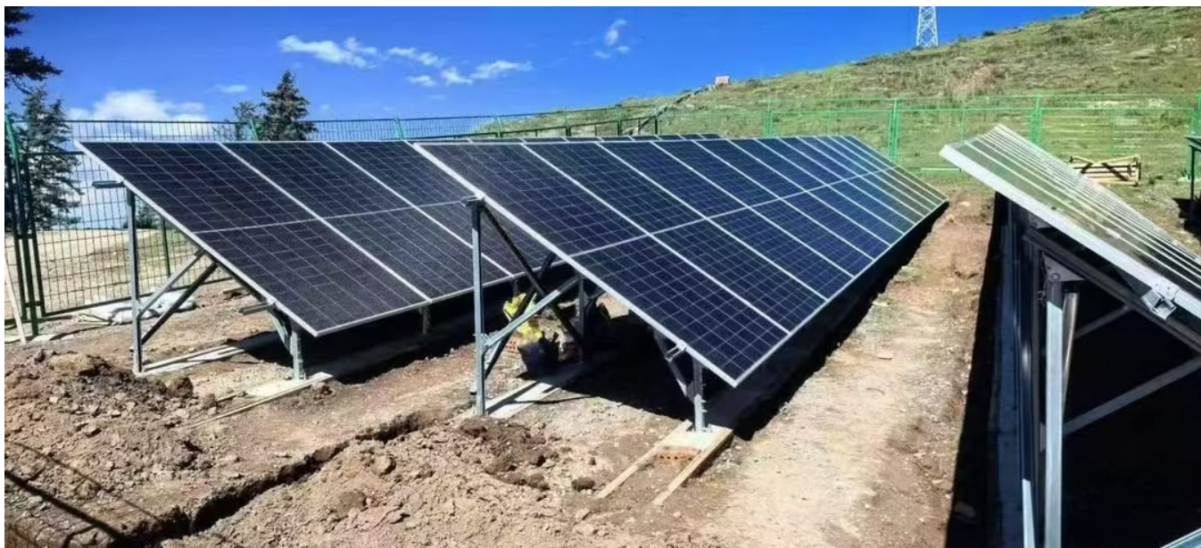
Reference: two-leg ground-mount tables of the type covered by this BOM.
