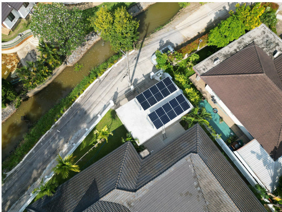
10 panels (6.500 kWp) on the carport roof, aerial view after installation.
